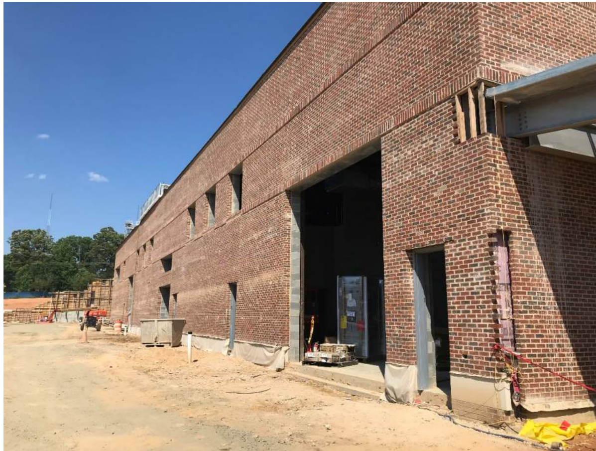
Overhead Roll Up Door Opening (131B) – SW Corner
