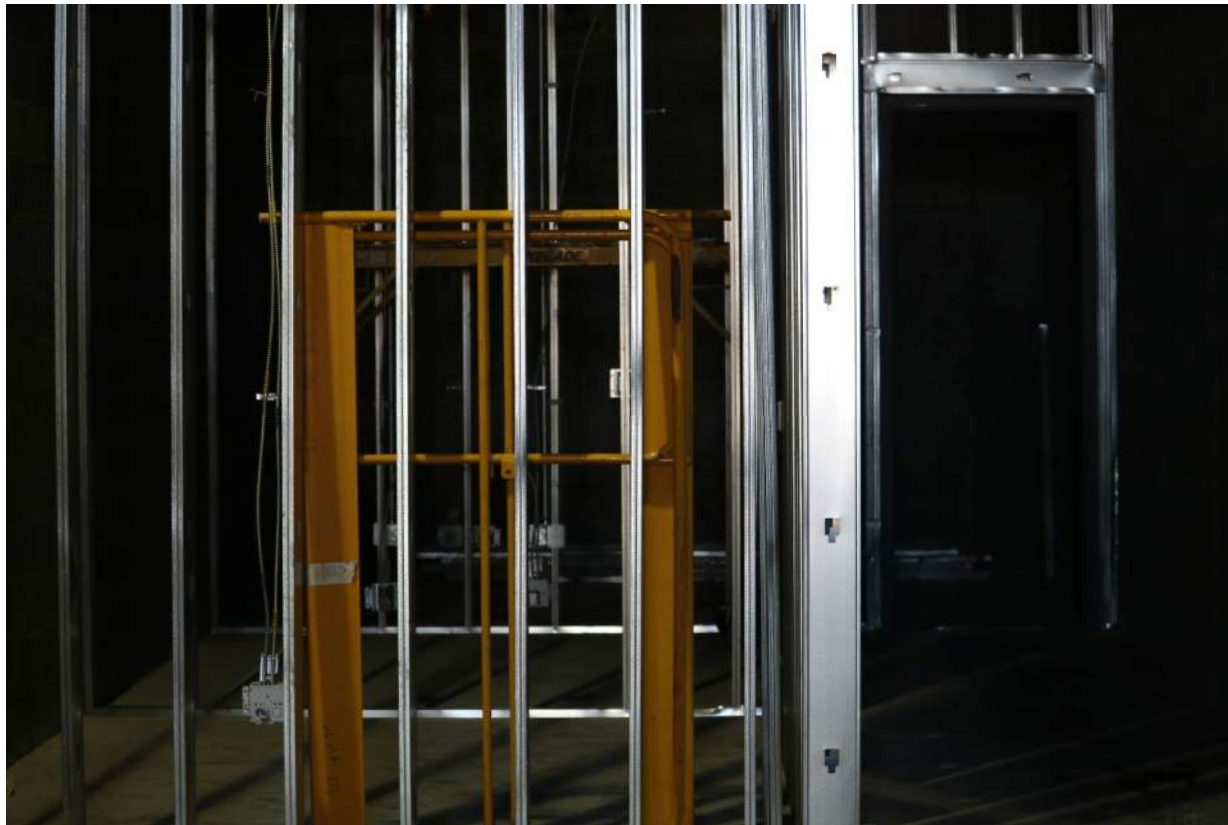
Framing of Welding Offices on Plaza Level
